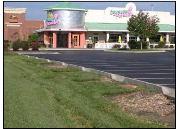
Impervious Area Disconnection. Photo Source: City of Kitchener, ON
