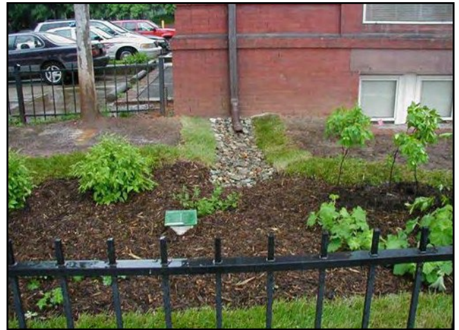
Rooftop Disconnection. Source: LID Center
