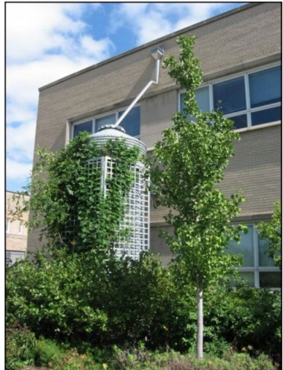
Distributed Site Design Measures, such as this cistern, can provide significant reductions in site runoff.
