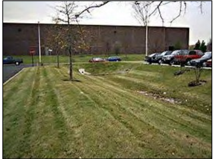
Grassed swale. Photo Source: EPA
