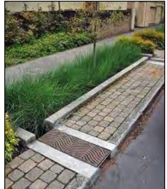
Roadside Bioretention. Source: sitephocus.com
